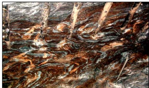
Figure 7. Anilio tunnel. Poor quality flysch (right bore at chainage 12+579)
