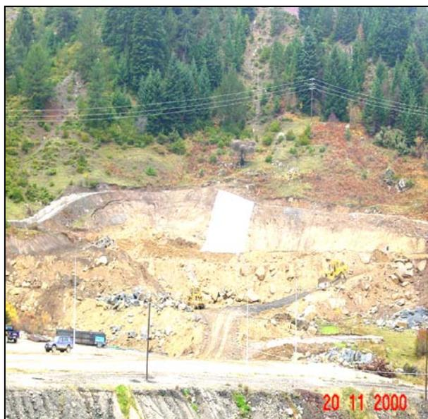
Figure 3. Landslide in the exit portal of Anilio tunnel
