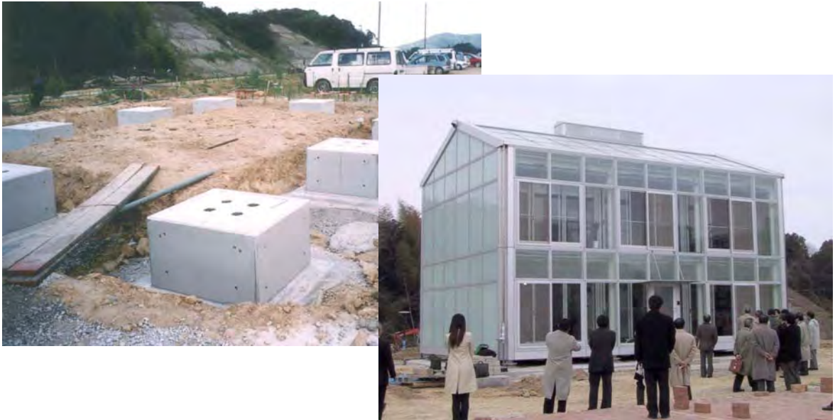
Precast Concrete Foundations Made from CRC in Kita-kyusyu
