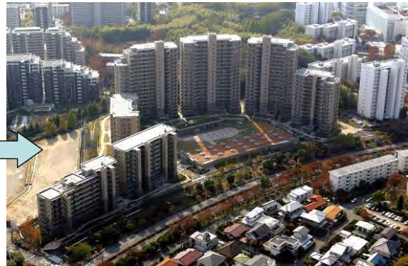
New apartment Houses 7 x 9-19-storied Recycled coarse aggregate: 3,000 t Recycled concrete volume: 3,000 m 3 ( Total concrete volume: 40,000 m 3 )
