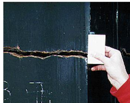
Signs of panel zone deformation
